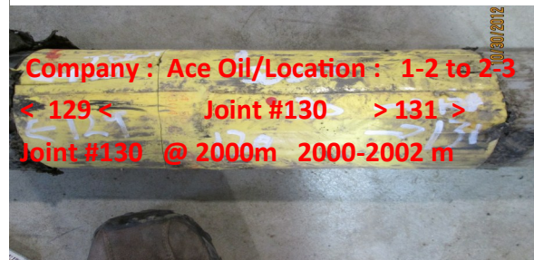
External View Starting weld with Location and Joint number and direction to next and previous Joint./ Section #
